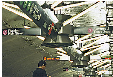
Functional stainless steel ceiling sculpture on 7 platform incorporating lighting, signage, LED, and fan system
